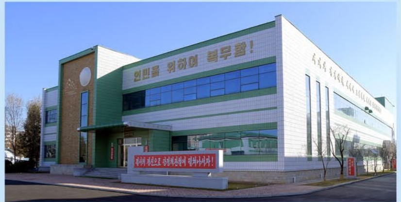
Newly-built Pyongyang Pharmaceutical Factory
